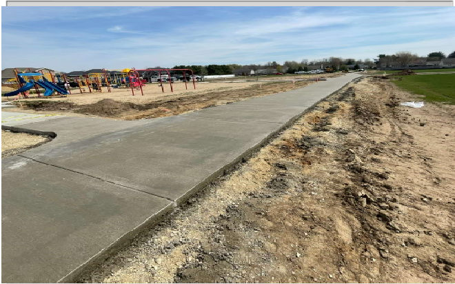
10' walk being poured on East side of park
