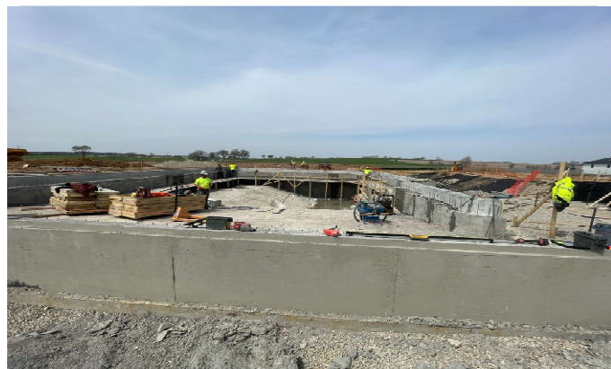
Second half of lap pool walls poured
