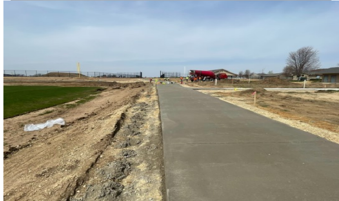
10' walk being poured on East side of park
