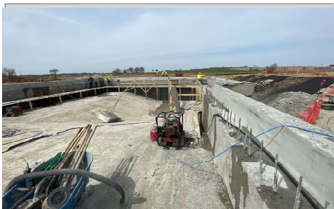
Second half of lap pool walls poured
