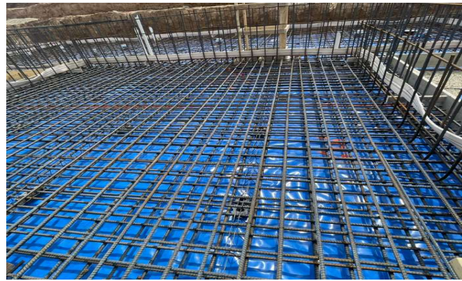
Surge tank room floor rebar installed
